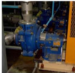
SH/50C 渣浆泵在氧化铝工厂 输送腐蚀性渣浆。 A SH/50C slurry pump handling hot caustic slurry in an alumina plant.
